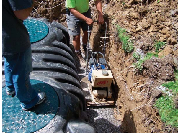
Photo 4.1.8-Example of mechanical compaction
