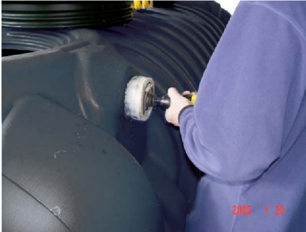
Photo 4.1.1-Drilling of inlet and outlet holes
