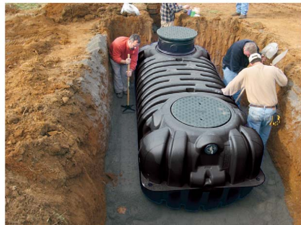
Photo 4.1.6-Spreading & compacting of backfill material
