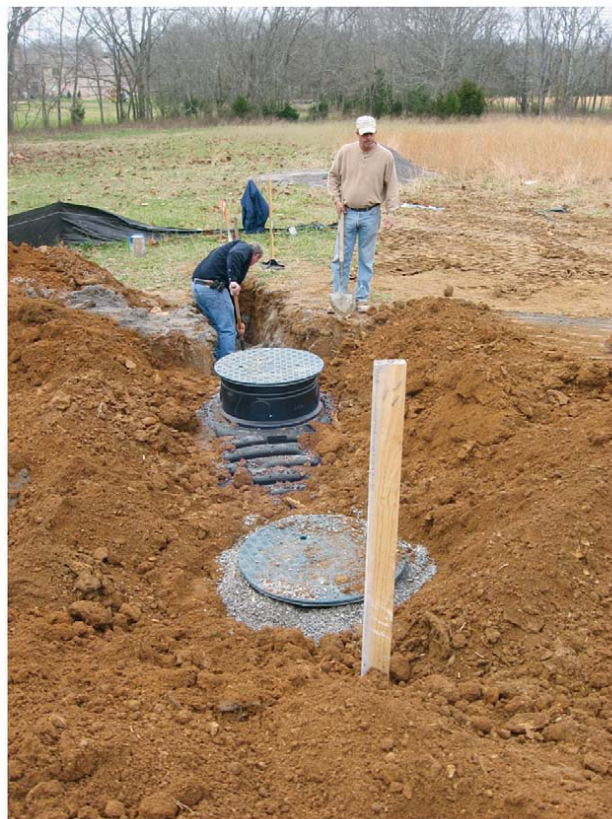
Photo 4.1.12-Example of complete backfill
