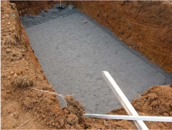
Photo 4.1.4-Bedding material prepared for setting the tank
