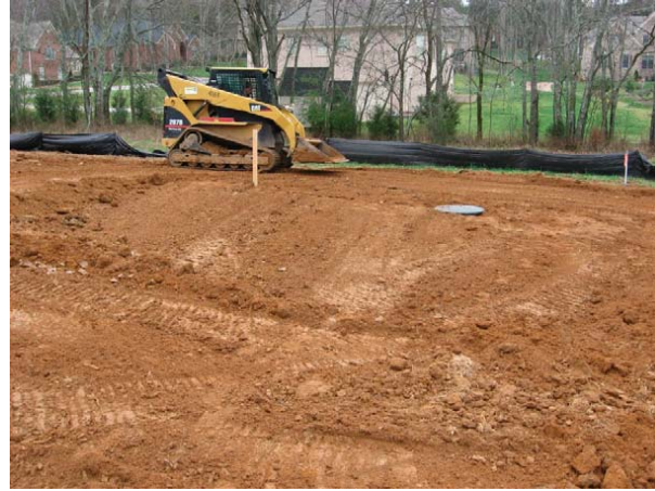
Photo 4.1.14-Example of final grading
