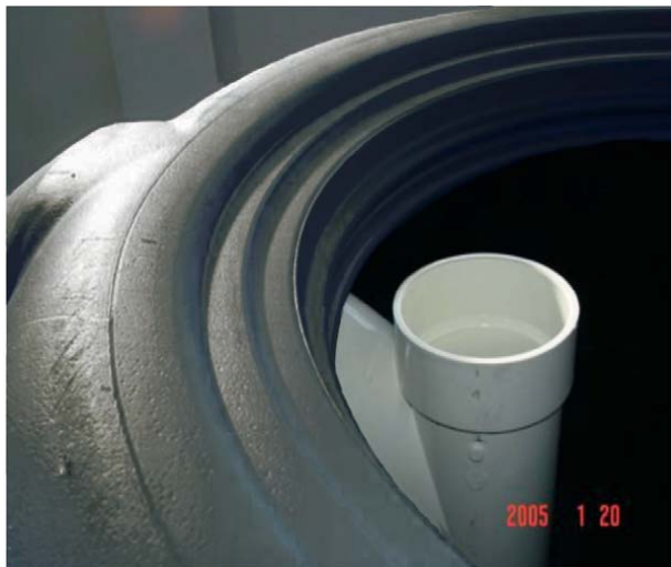
Photo 4.1.16-Pipe located inside the edge of the manway
