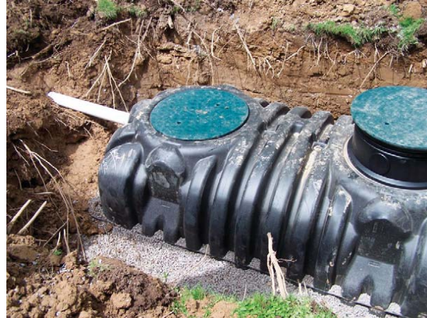
Photo 4.1.9-Uniform level distribution of material
