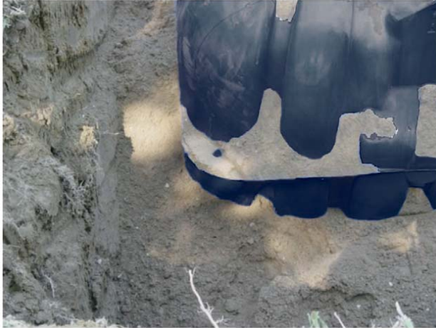
Photo 4.1.7-Proper support for vessel
